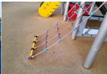
**Finding:** The rope anchor bar forms a hard object within the **Action:** Monitor - No remedial work recommended falling space of the equipment in contravention of the requirements of BS EN 1176 Part 1
