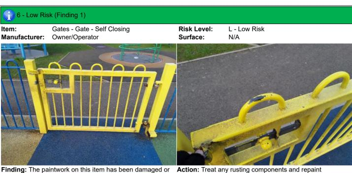
worn exposing the metal underneath which is rusting
