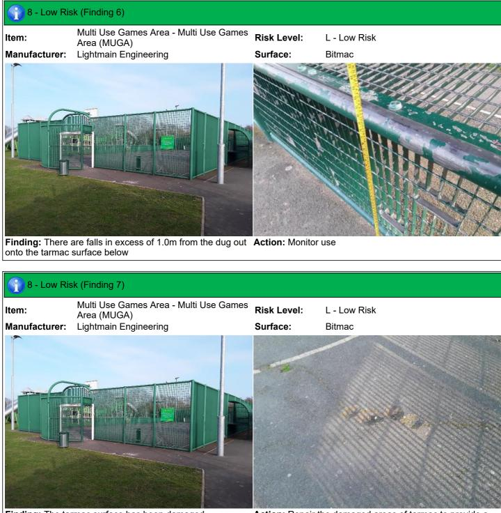
Finding: The tarmac surface has been damaged
