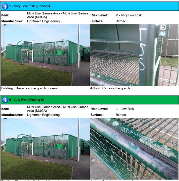
Finding: The paint is flaking off the metalwork
