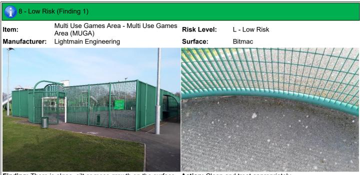
**Finding:** There is algae, silt or moss growth on the surface **Action:** Clean and treat appropriately resulting in slippery conditions
